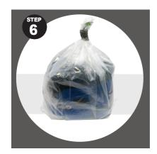
Place the extractor into a 200UM clear bag and tape using duct tape. Repeat this process twice.
